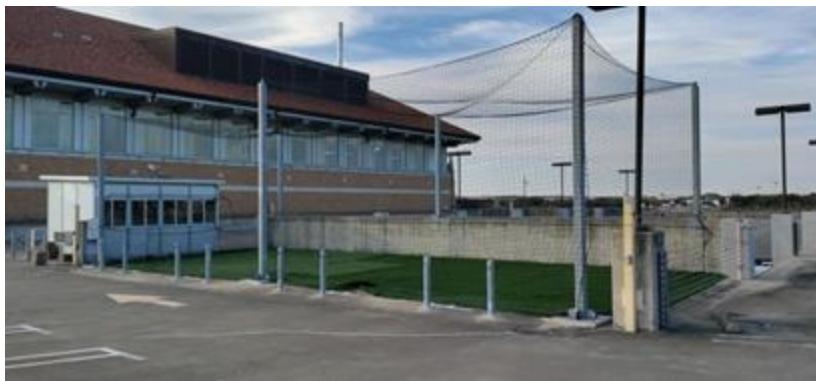
Radionavigation Lab Rooftop Drone and Satcomm Facility
